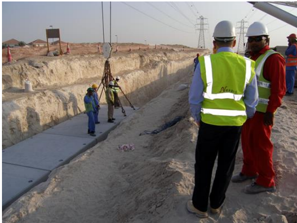
Construction of cable tunnel (cut and cover method)
