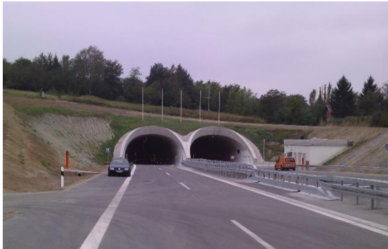
East portal of the Leutenbach tunnel
