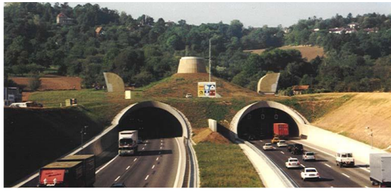
North portal of the Engelberg tunnel
