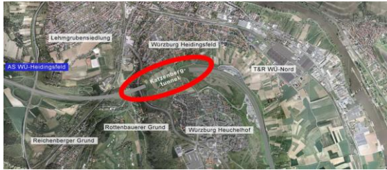
Location of Katzenberg tunnel near Würzburg on A3 federal highway (from: V-KON.media GmbH)
