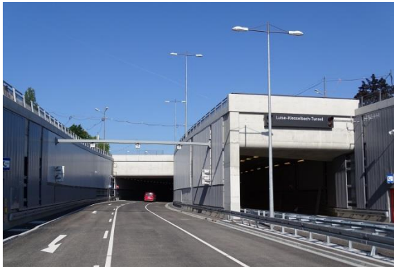
South portal of the Luise-Kiesselbach-Tunnel
