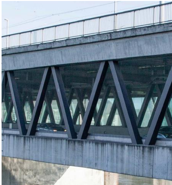
Bearing structure of the Dreirosenbrücke
