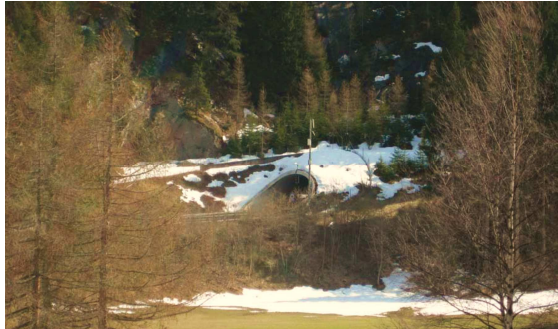
Tunnel Bärenburg on alpine location
