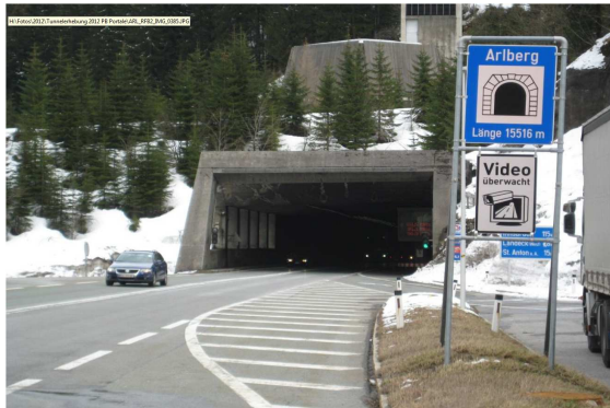
With 15,516 m, the Arlberg Street Tunnel is one of the longest road tunnels in Europe
