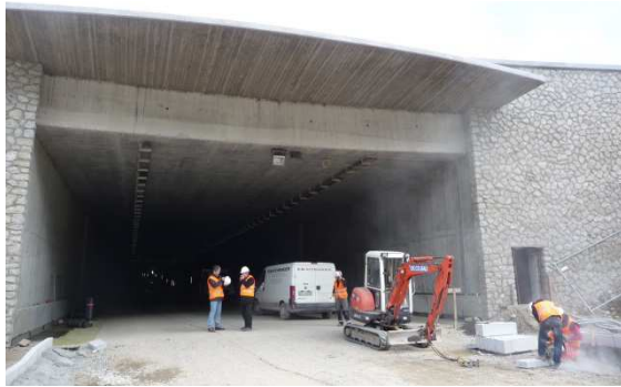
Tunnel portal Mebo
