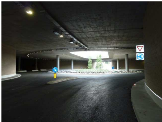
Underground roundabout, exit to the railway station
