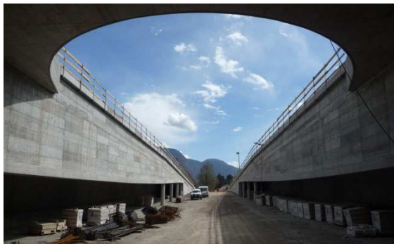
Entry and exit ramps at the railway station Meran
