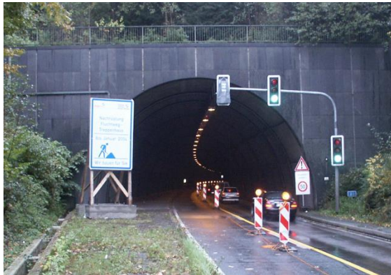
Eastern tunnel portal into the lower tube
