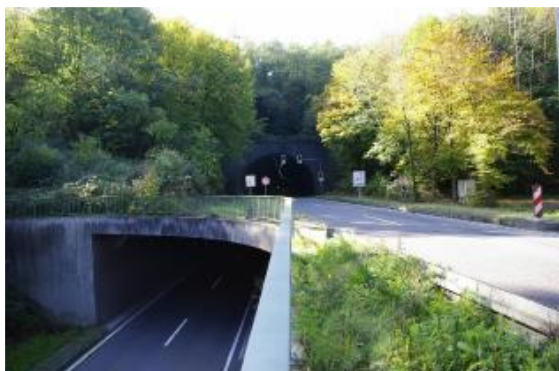
Western tunnel portal with two traffic tubes in vertical arrangement
