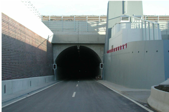
Weser Tunnel western portal
