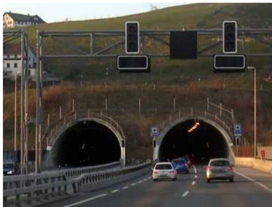
Uznaberg tunnel portal
