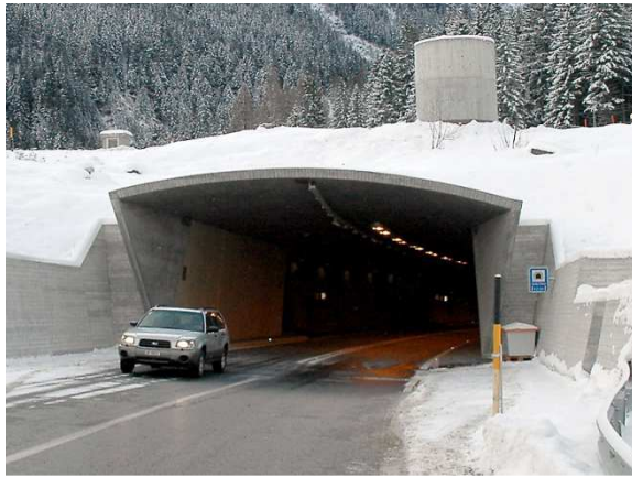
Tunnel Portal with exhaust stack
