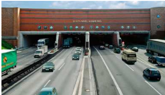
Northern Portal of the Elbe Tunnel with 4 tubes
