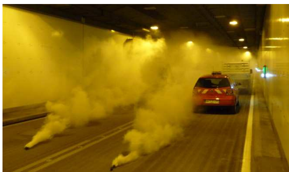
Smoke test during ventilation system commissioning
