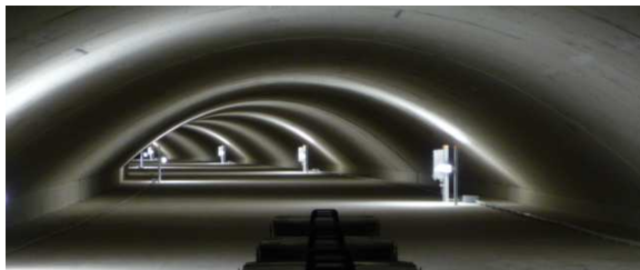
Exhaust duct after refurbishment
