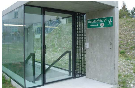
Emergency exit on the outside
