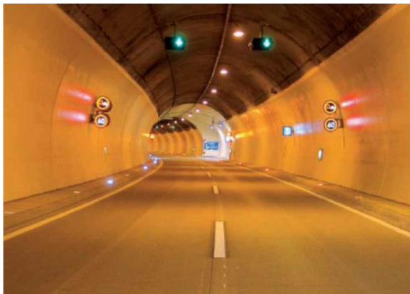
Traffic space of the Ambergtunnel after renovation
