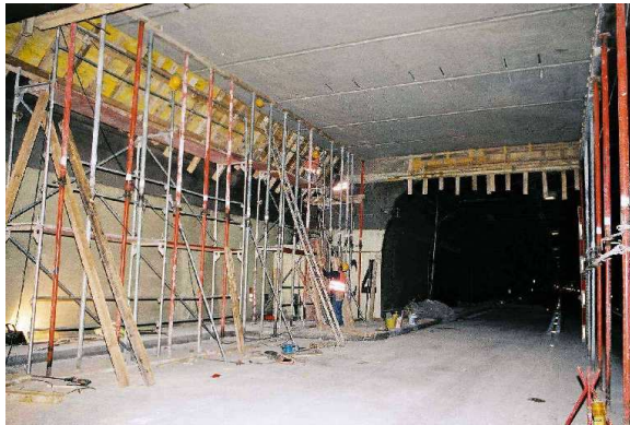
Construction of jet fan niches in the false ceiling
