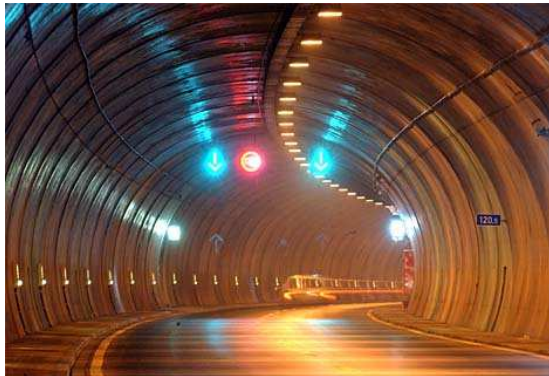
Check of the self-rescue measures in an existing tunnel
