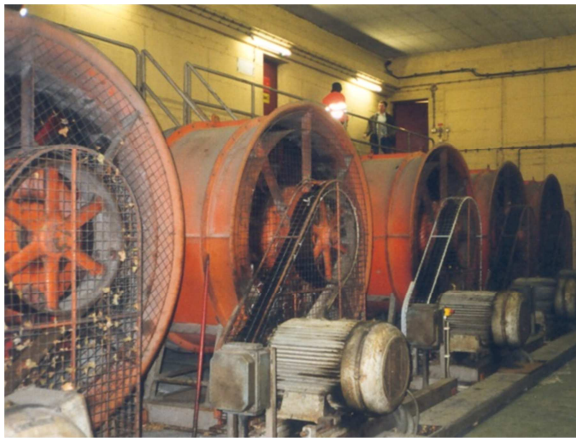
Fresh air ventilators before the refurbishment
