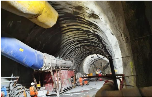
Tunnel environmental conditions during construction are affected by numerous factors
