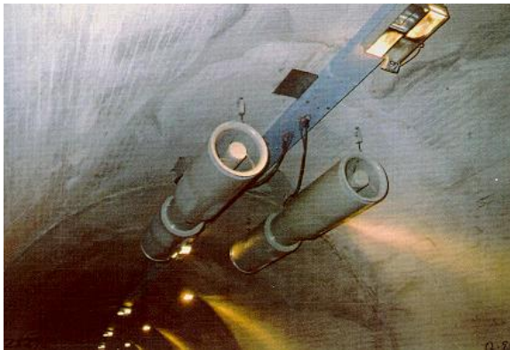
Installation and supply of jet fans
