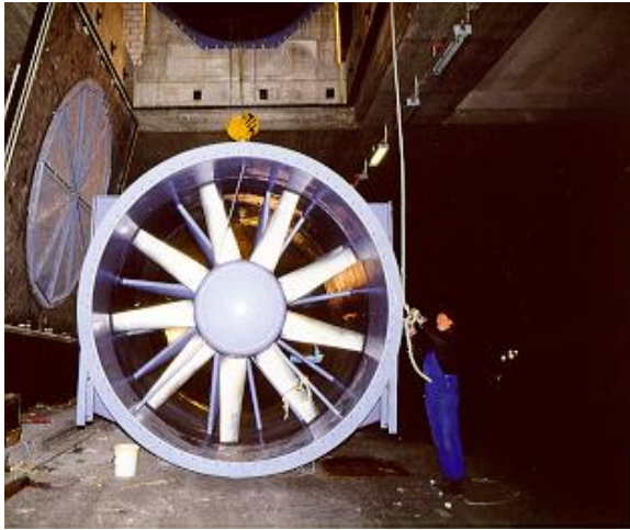
Mounting of an axial fan
