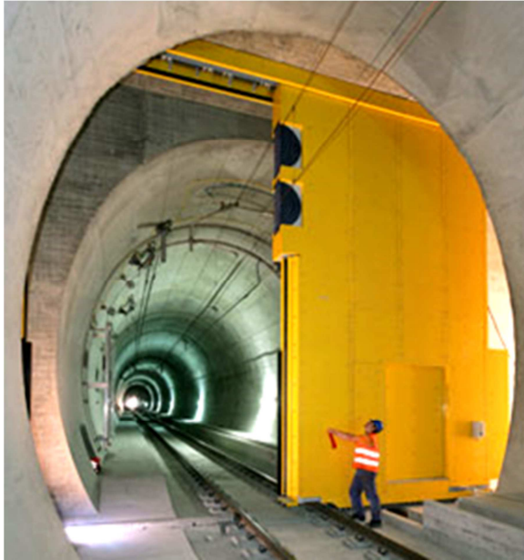
Door in rail tunnel
