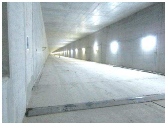
Structural works of tunnels of the Lusail LRT.
