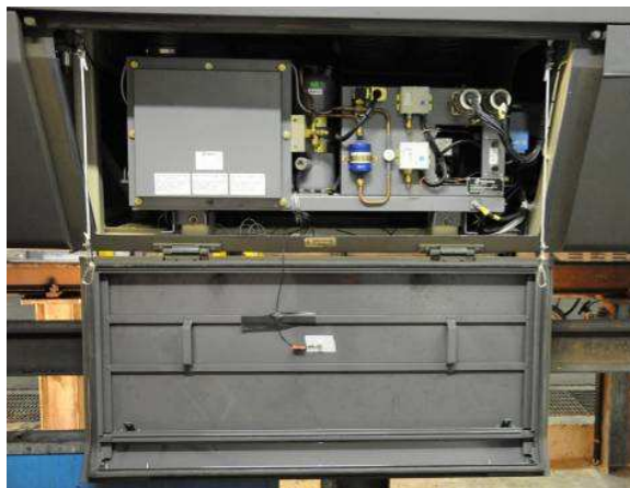
Assembly of a pressure transducer in a switch box
