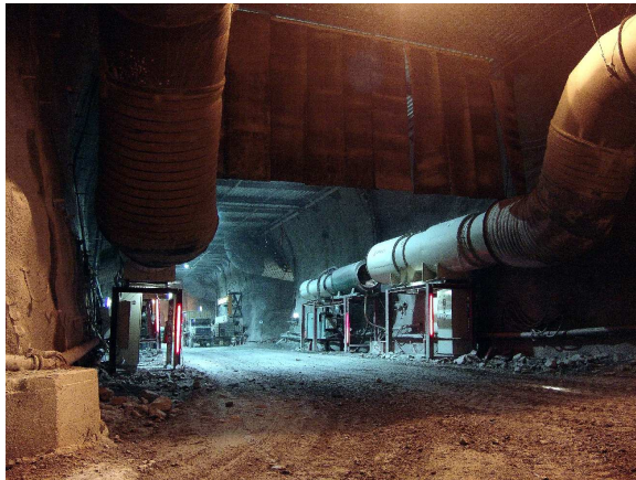
Application of air ducts, fans and air coolers during construction
