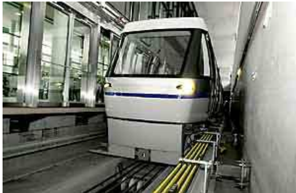
Skymetro in der Station
