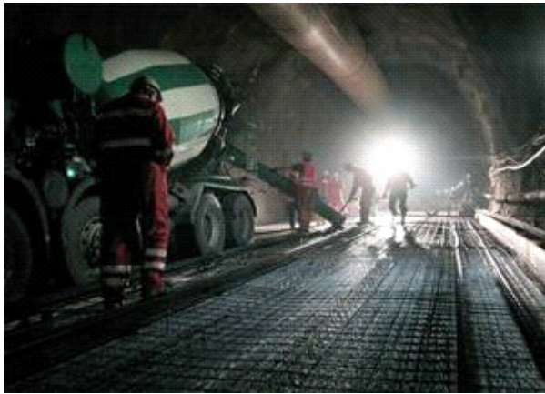
Construction of the trackway with preliminary ventilation
