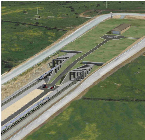
South portal of Guadarrama Tunnel
