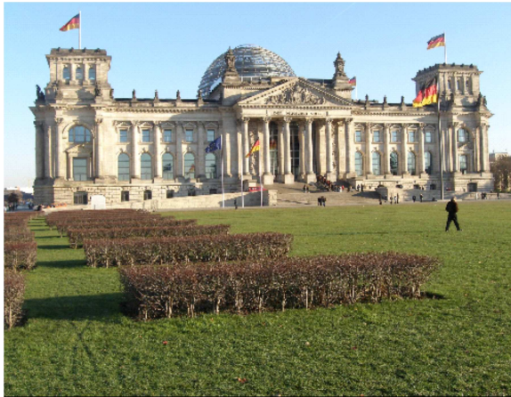
Underground line U55 passes below park in front of Reichstag building, Berlin
