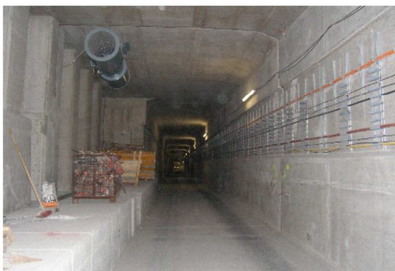
Jet fans for longitudinal ventilation of construction sites in tunnels and stations
