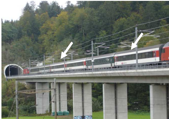
Test train with measurement equipment entering the Tunnel Murgenthal; positions of pressure transducers are indicated
