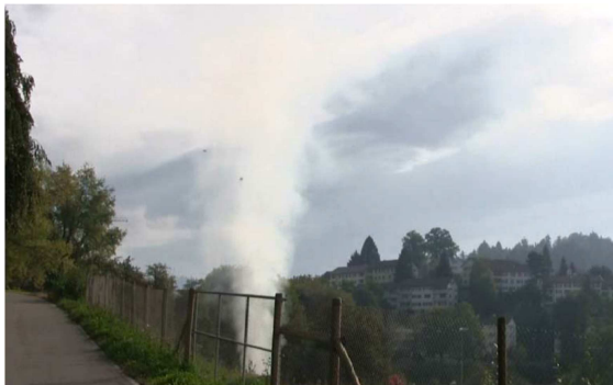
Smoke egress at the exhaust chimney
