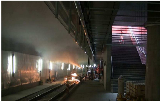
Fume layer East side with stairway
