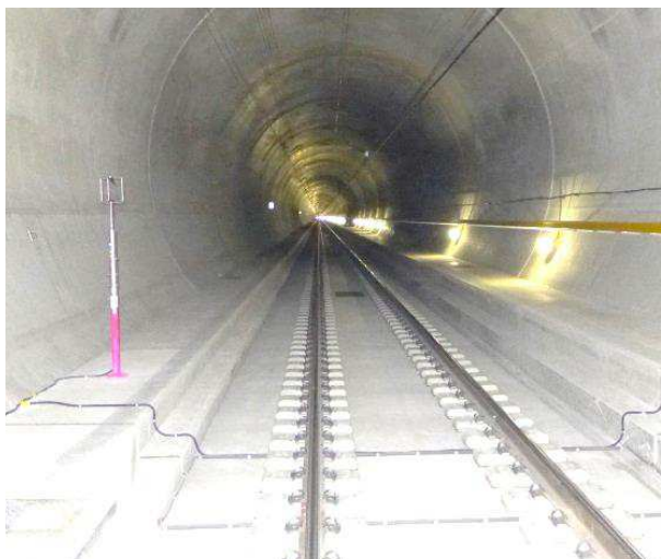
3D flow measuring system for assessing the air flow on the tunnel sidewalk during train passage
