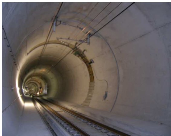
Single track tunnel: eastern tube
