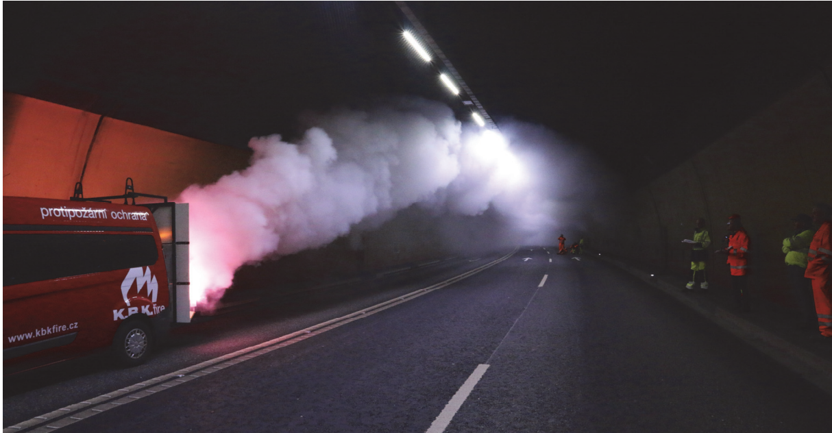
Figure 4: Moving smoke source in the Crapteig tunnel
