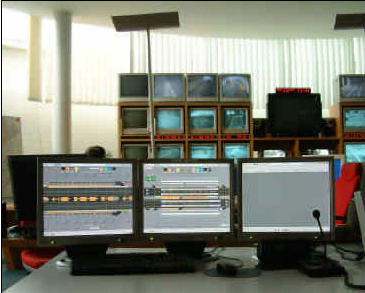
**Figure 5: Man-machine interface (MMI)**
