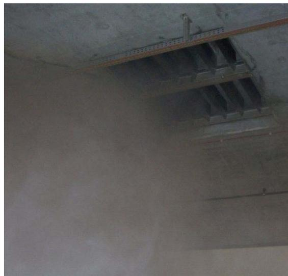
*Fig. 15 Non-toxic smoke extracted through the extraction damper in the Flüelen tunnel (Switzerland)*
