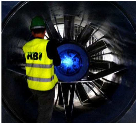
Main filtration fan: installation check
