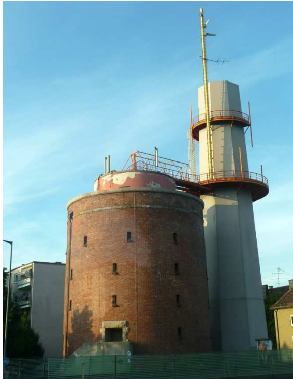
Exhaust stack at western tunnel portal
