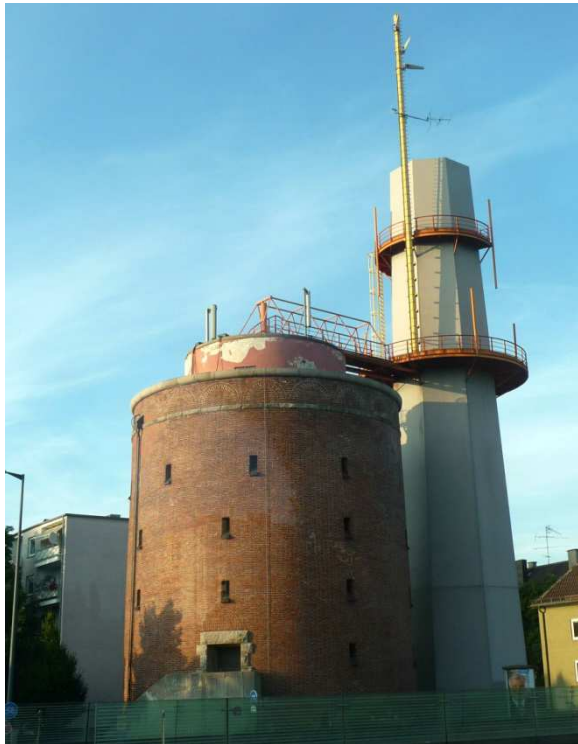
Abluftkamin am Westportal
