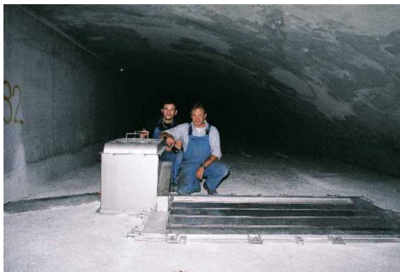
Mounting of a damper
