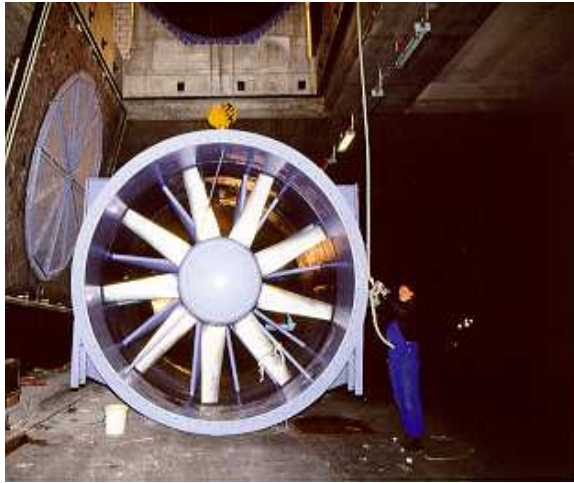
Mounting of an axial fan
