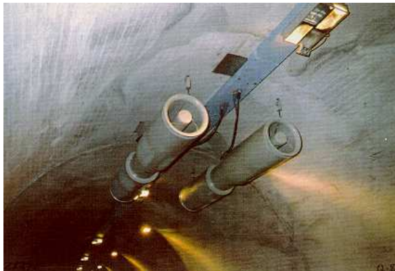
Installation and supply of jet fans
