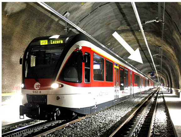
Jet fans of the emergency ventilation at the passover south (white arrow)
