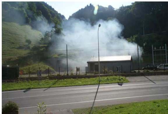
Smoke at the southern portal during a fire test
