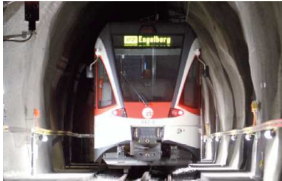
Passenger train in the Engelberg railway tunnel
