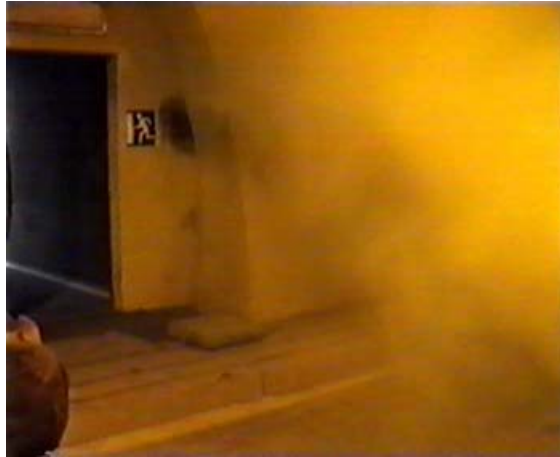
Fig. 13 Open emergency exit in the smoke zone. The escape route is entirely being kept free of smoke.
