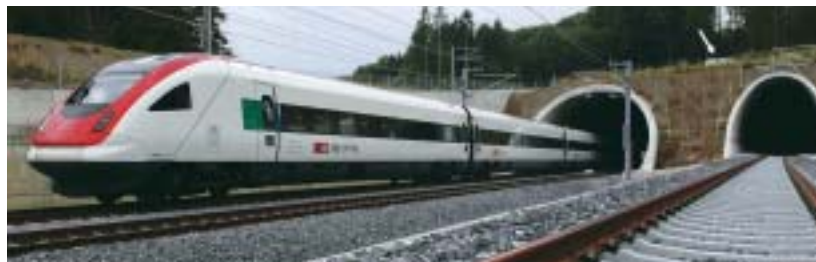
More extreme pressure fluctuations in single-track than in double-track tunnels; white arrow indicates pressure relief shaft
