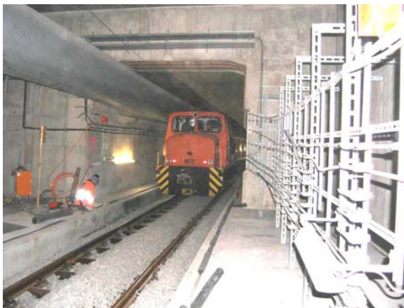
Air ducts in tunnel along trackway with locomotive during installation works
